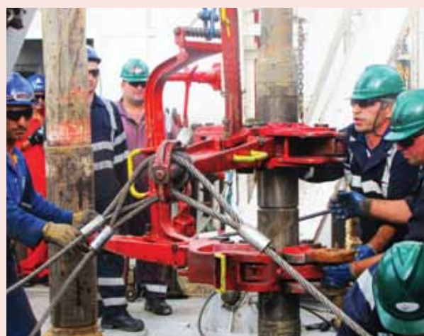
Figure 2 – Drilling operations – Mukhiani #1 Well
