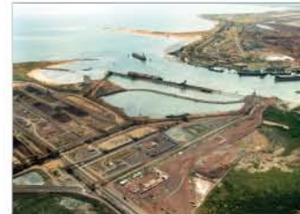
Landside Marine Infrastructure
