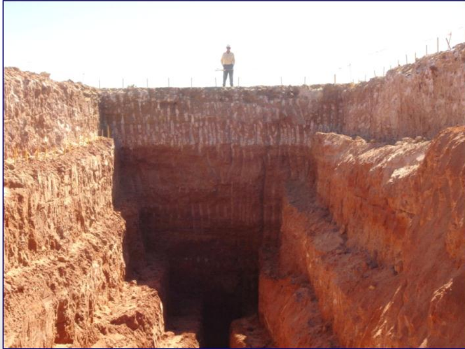
Trench for Bulk Sample
