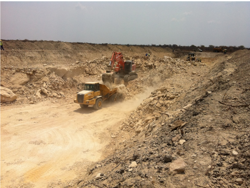
Diagram 4 Removal of overburden from the first blast with a 50t digger.
