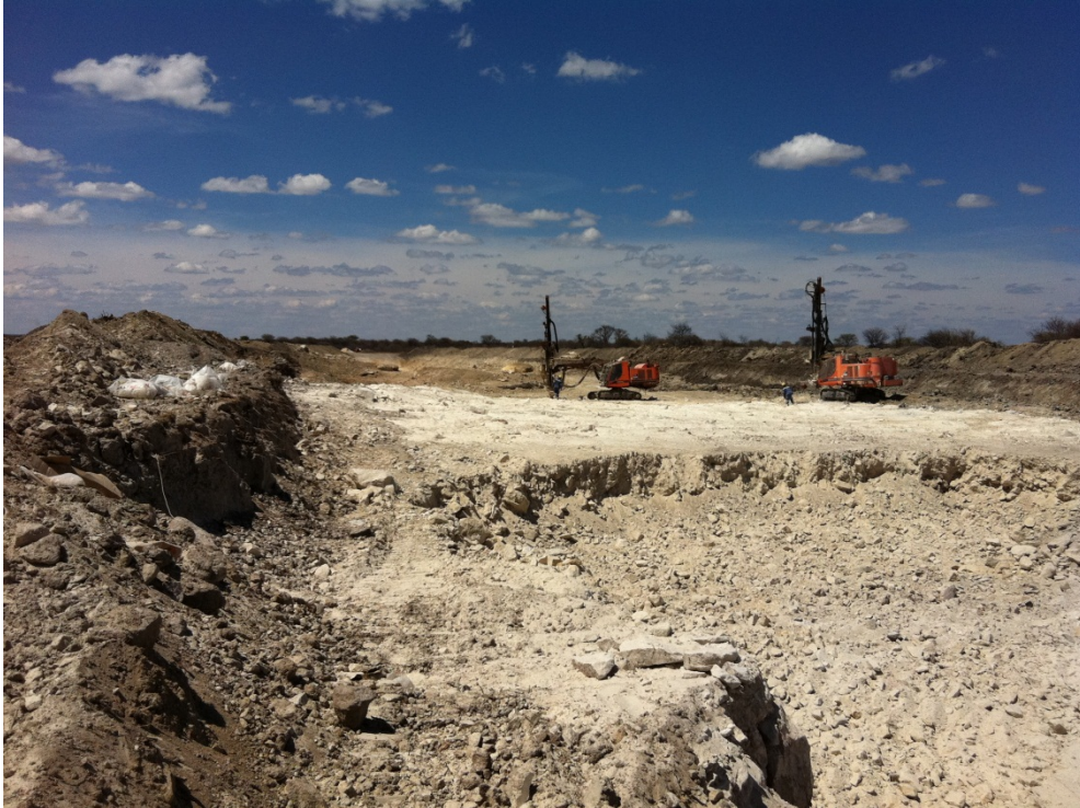
Diagram 3 Blast-hole rigs drilling overburden on the first blasting bench.
