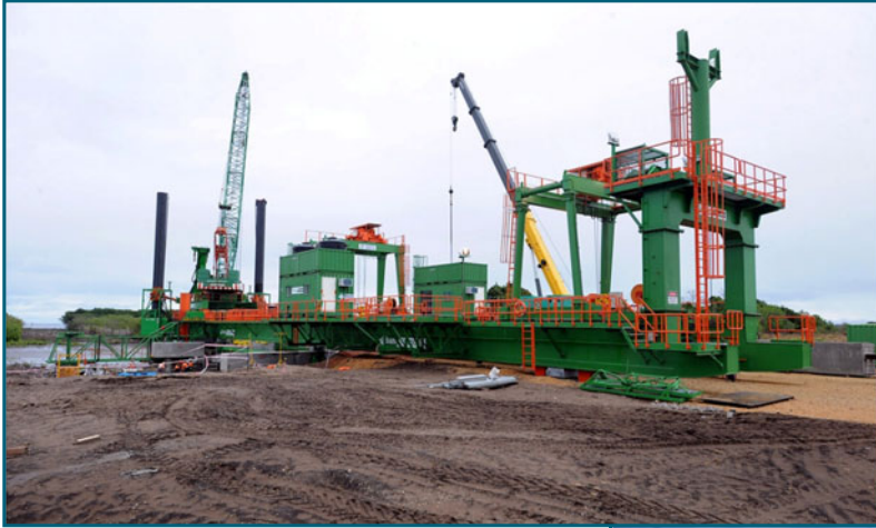
Marine jetty piling
