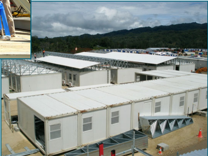
Hides Gas Conditioning Plant - Pioneer camp construction
