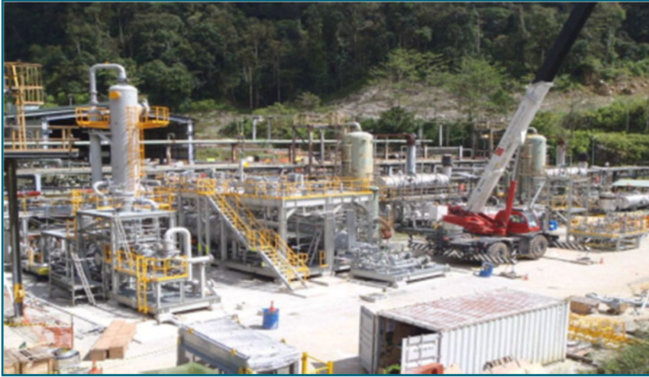
TEG Dehydration Unit installation
