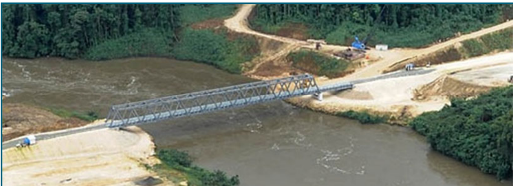
Completed Mubi River crossing
