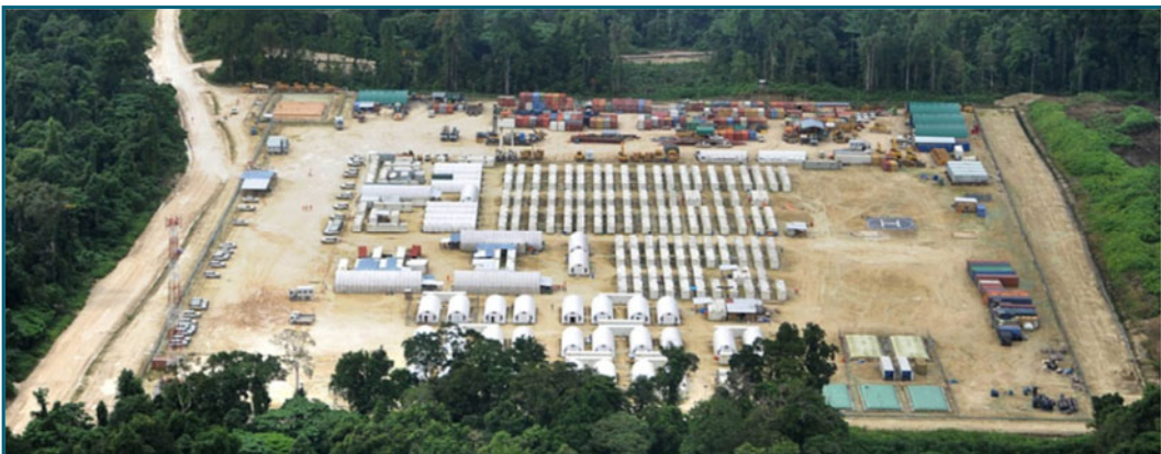
Kopi Scraper Station
