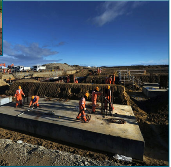
Process pipe rack construction
