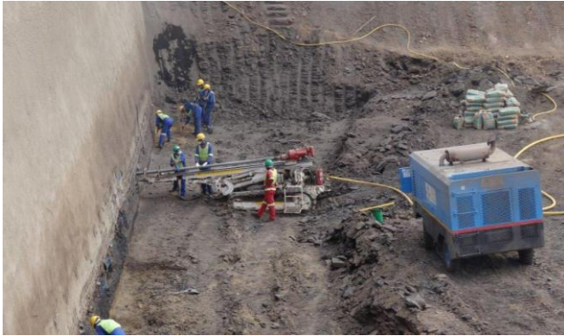
Support work on the highwall of the portal
