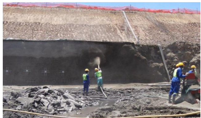
Support work in the Penumbra Coal Mine box-cut with soil nails, wire mesh and shocrefing work
