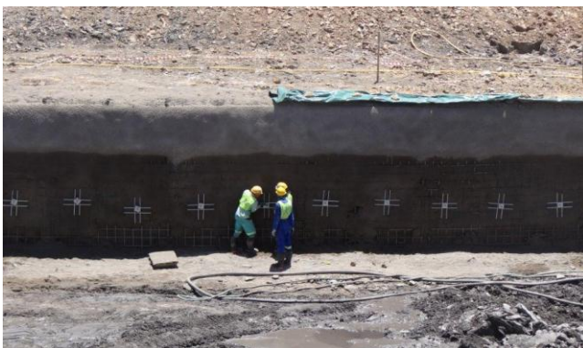
Support work in the Penumbra Coal Mine box-cut with soil nails, wire mesh and shocrefing work
