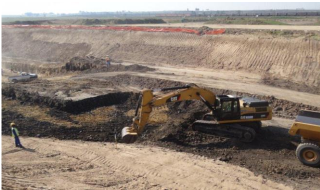
Excavation of the ramp in the box-cut
