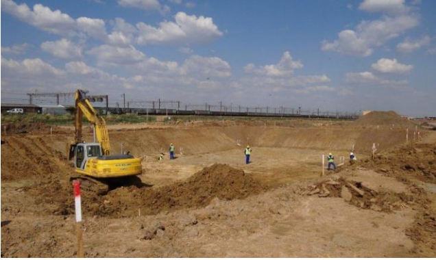
Civil works for the pollution control dam have been completed and lining of the dam has now commenced
