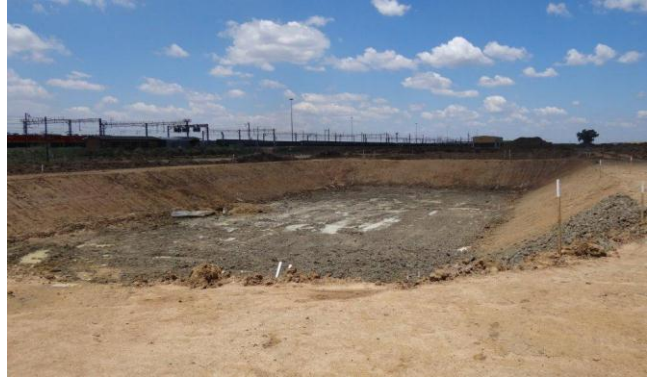
Civil works for the pollution control dam have been completed and lining of the dam has now commenced
