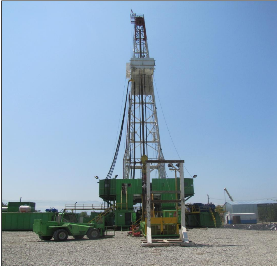
Drilling operations on the Mukhiani 1 Well
