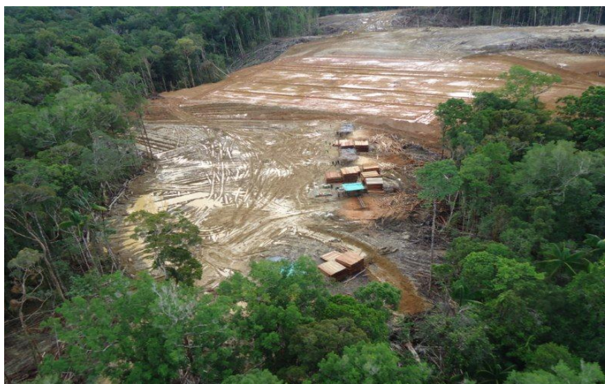
Ketu-2 wellsite being prepared for drilling as at 5 December 2011
