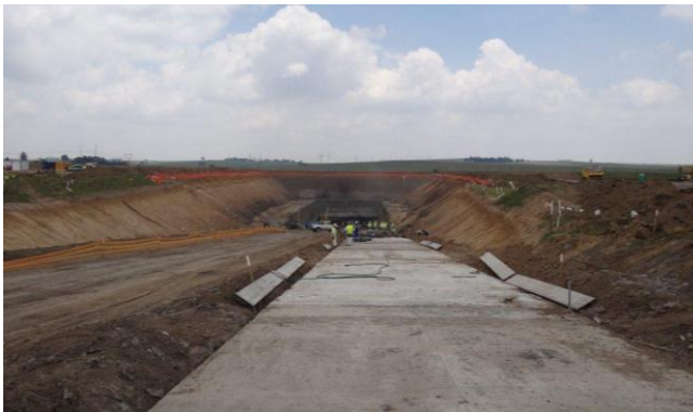
Construction of the concrete access ramp into the Penumbra Coal Mine box-cut
