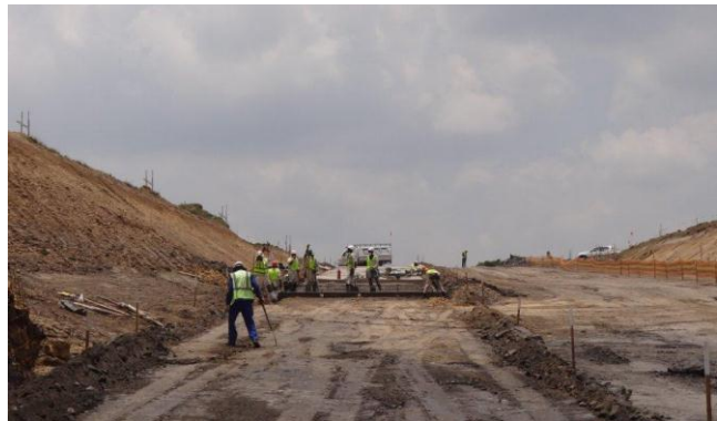
Construction of the concrete access ramp into the Penumbra Coal Mine box-cut
