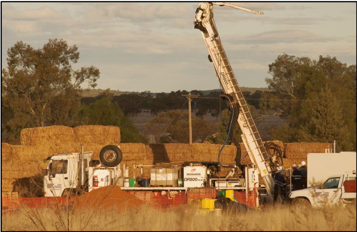
Deep drilling – Nymagee Copper Mine
