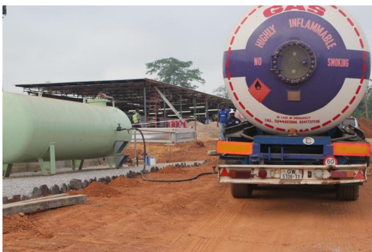
Initial gas delivery enabling commissioning to commence
