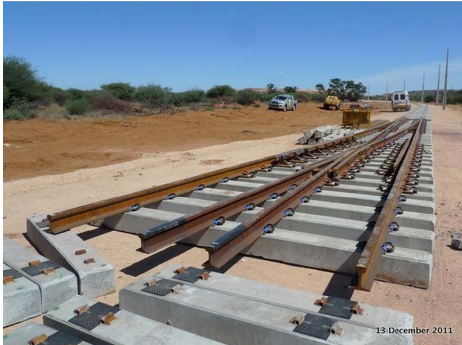
Rail siding sleepers in place and rail fastening installation commenced
