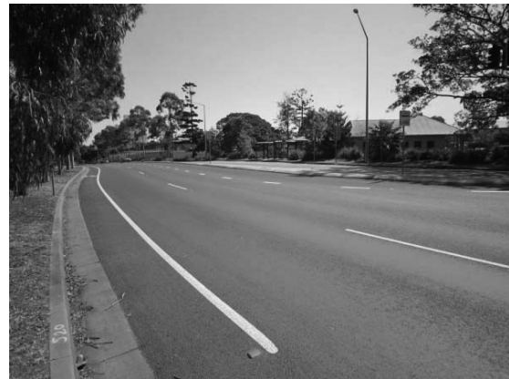
VIEW WEST ALONG HOLKER STREET
