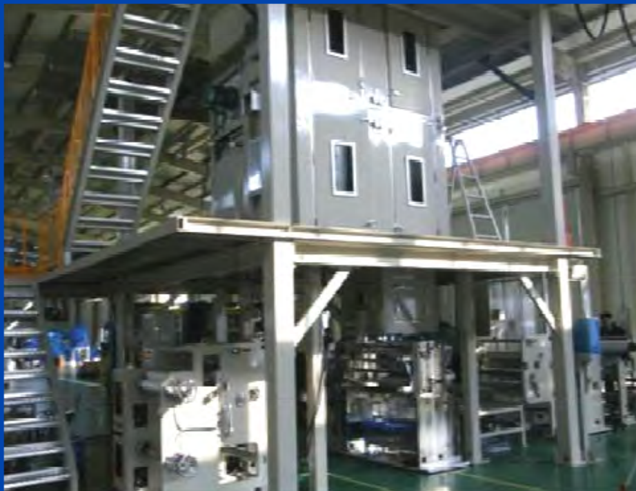
KUBT separator formation machinery
