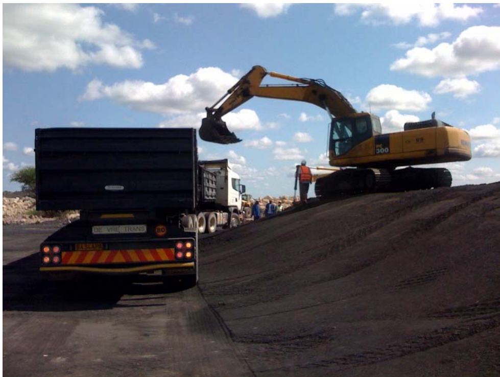
Diagram 7 Coal from compacted stockpile being loaded onto road train for shipment to processing facility in South Africa.
