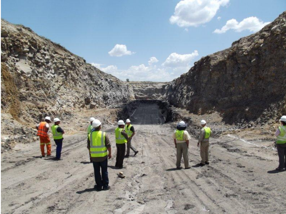
Diagram 6 Bulk sample excavation status in mid-January, ready for final drilling and blasting of Lower Main Seam coal.
