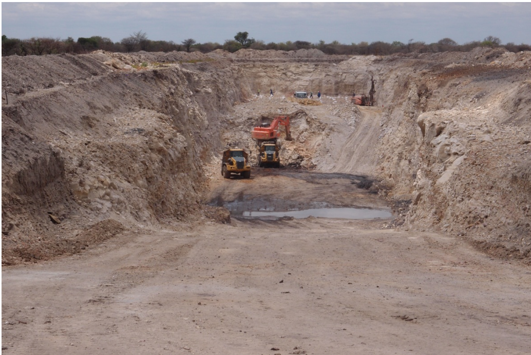
Diagram 3 Drilling and blasting of the final waste rock (overburden) in late November 2011
