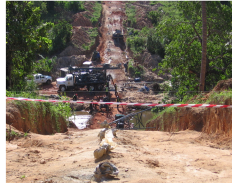
Mukurumudzi Dam wall foundation grouting
