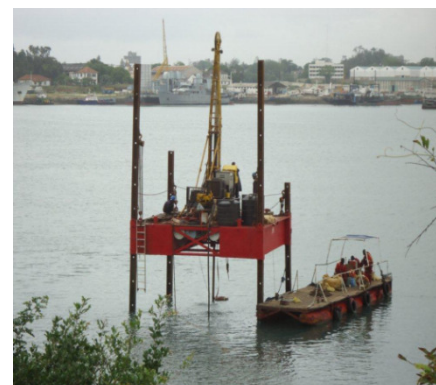
Port geotechnical drilling
