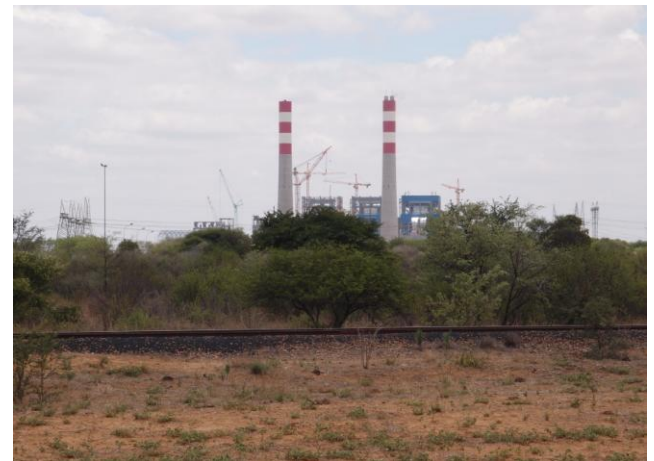
Morupule B (4 x 150MW) under construction
