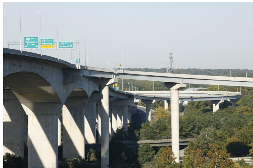
Pocahontas Parkway: James River Bridge
