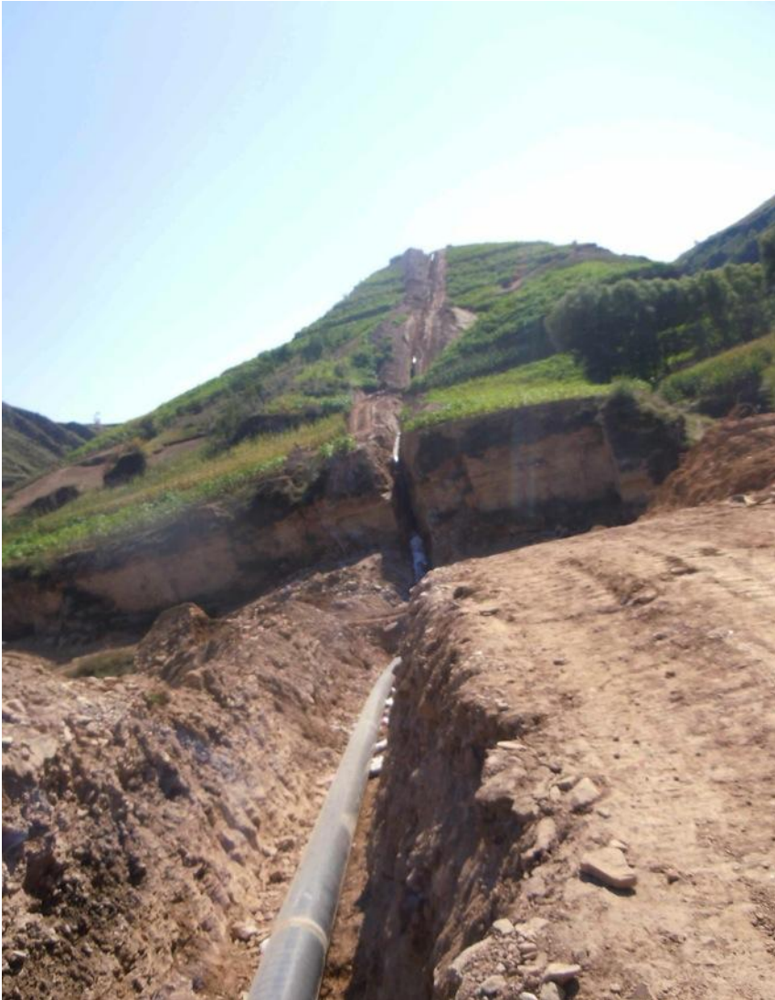
Pipelines traversing Sino Gas's PSCs under construction
