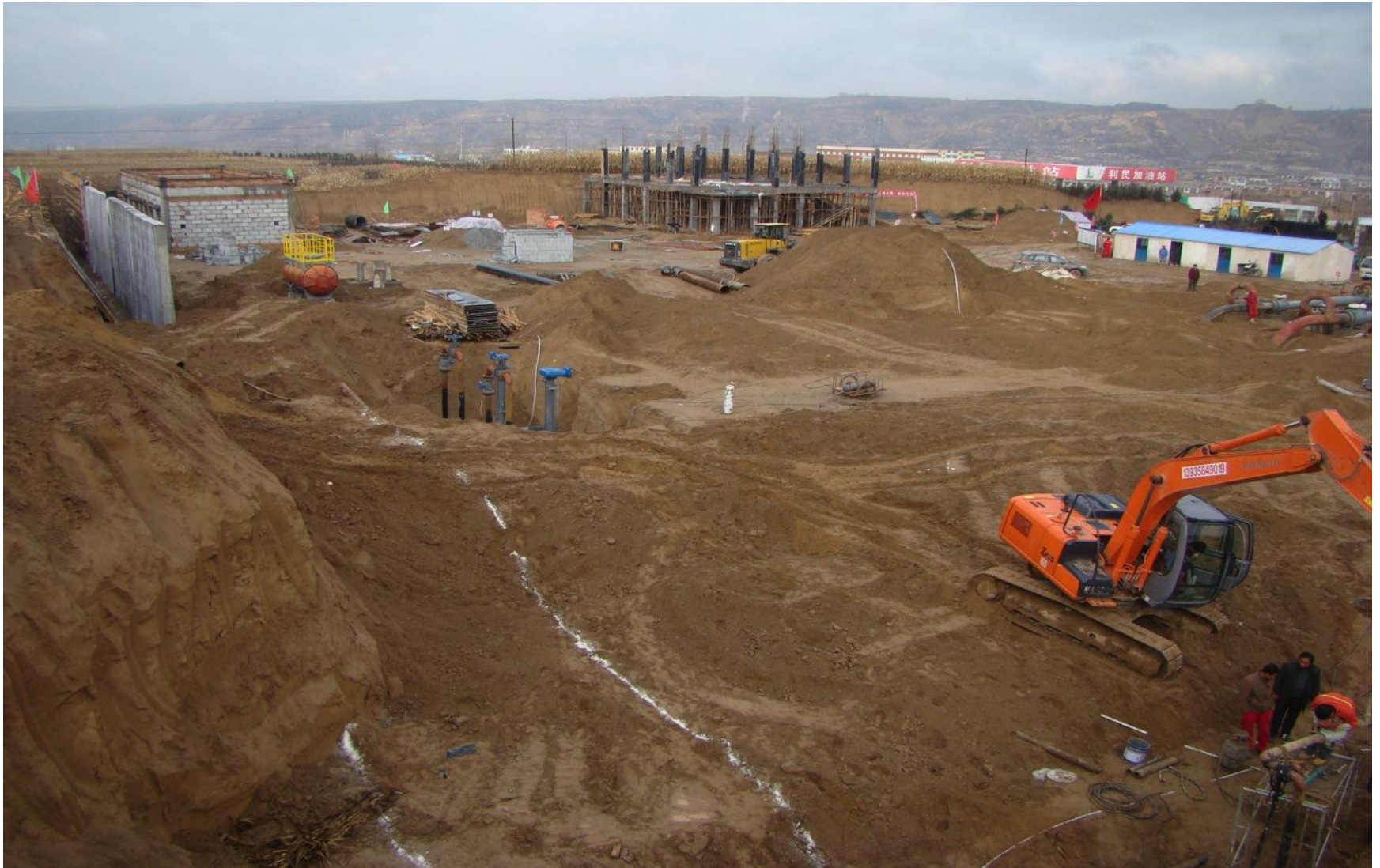
Gas processing facilities under construction in Shanxi province
