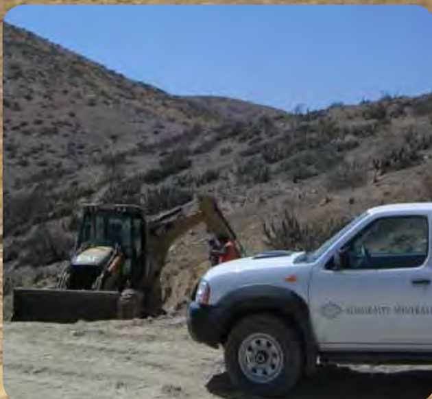
Excavator preparing platform for an up to 600 metres deep drill hole at La Chulula.
