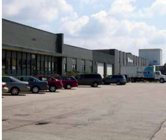
1900-2060 PRATT BOULEVARD, CHICAGO, ILLINOIS, USA
