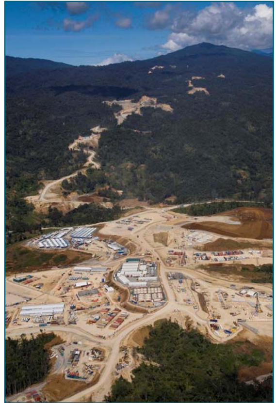
HGCP & Hides spipeline road
