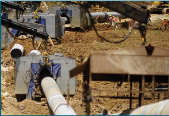
Pipe welding team
