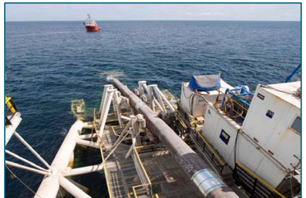
Offshore pipelay – SEMAC I
