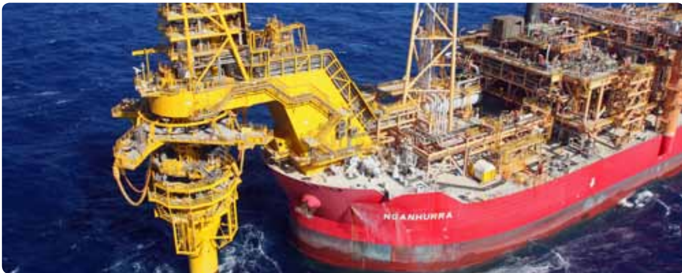
The Nganhurra FPSO, in offshore Western Australia, gathers, stores and offloads crude oil that has been produced from Enfield oil field.
