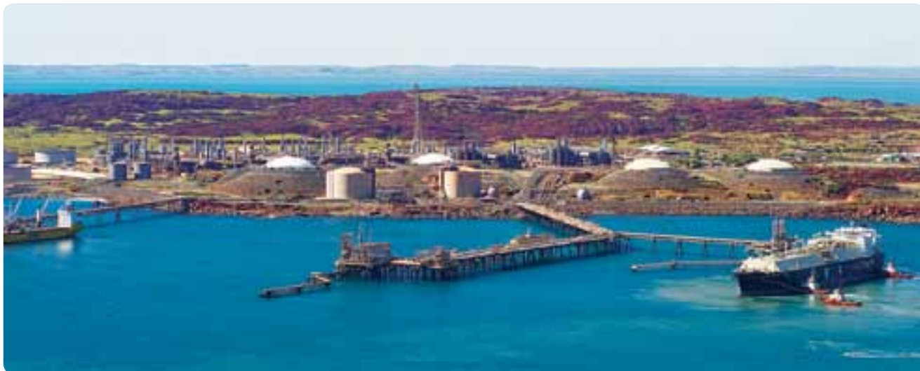
Woodside Donaldson LNG vessel arrives at the NWS Project Karratha Gas Plant to receive its LNG cargo for transport to overseas markets.
