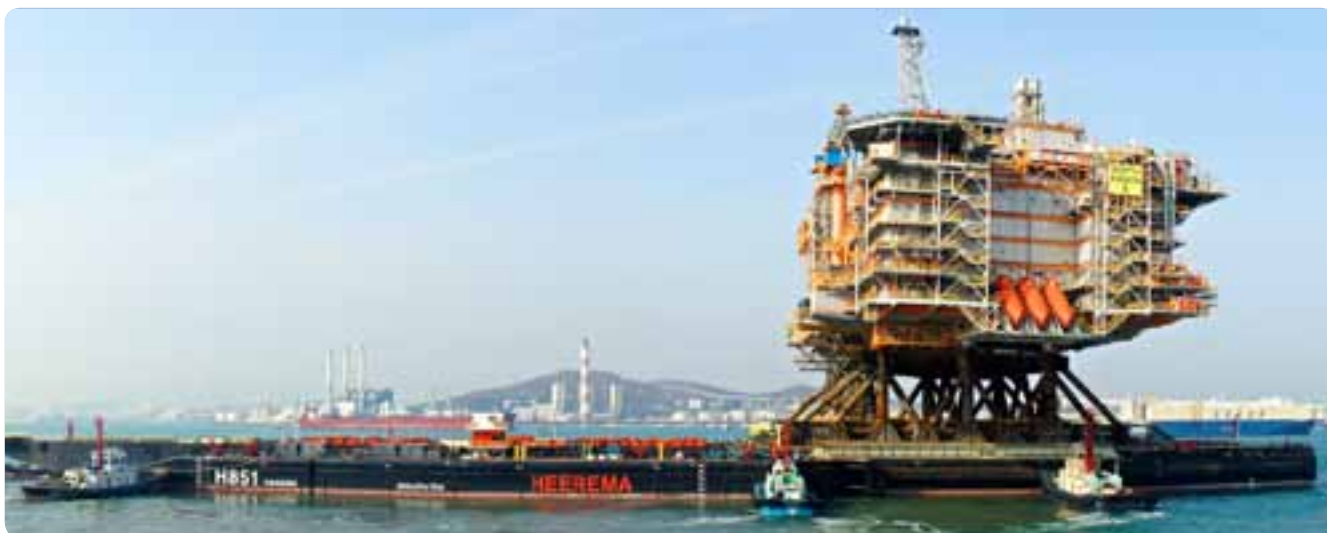
North Rankin B topsides on the heavy lift 'Heerema' barge, commences the journey from the Republic of Korea construction yards to the North West Shelf.
