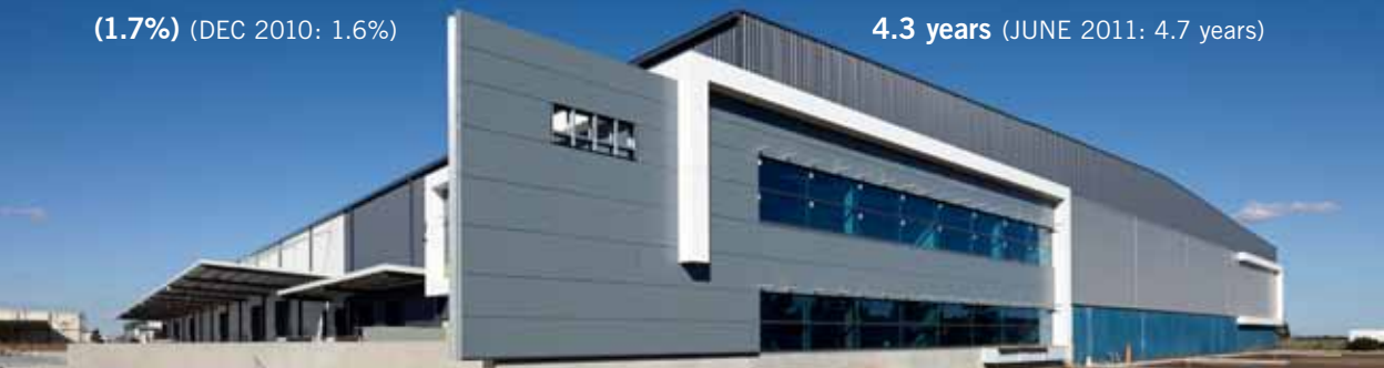
Spec development, 2-10 Distribution Drive, Laverton North, VIC
