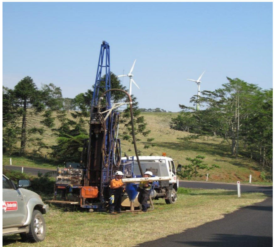
Figure 6 Ravenshoe East Drilling
