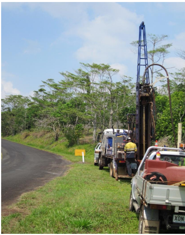
Figure 5 – South Johnstone Drilling
