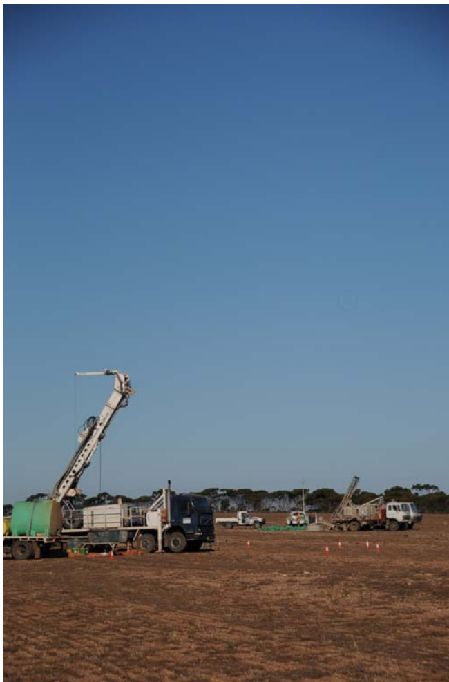
Plate 1: Two drilling rigs at the Paskeville Prospect.
