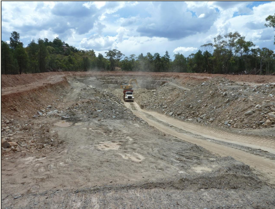
Hera Boxcut – 18 th Feb 2012
