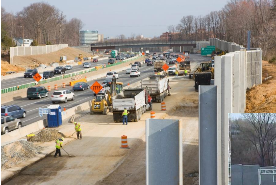
Late 2010: Outer lane construction view
