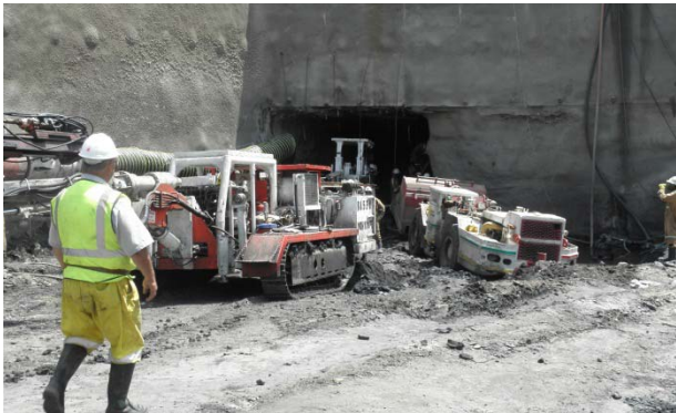
Activities at the entrance to the twin declines in the Penumbra Coal Mine box-cut
