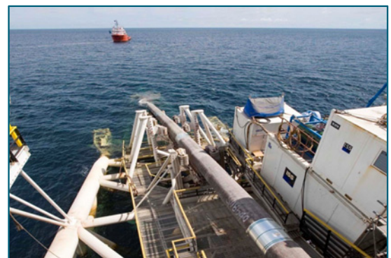
Offshore pipelay – SEMAC I
