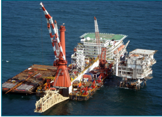
Pipelay Barge 'Lewak Champion' along side Kumul Terminal
