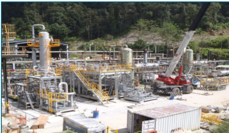
TEG Dehydration Unit installation
