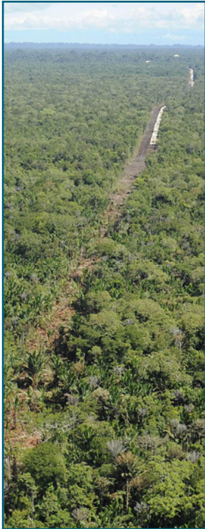
Pipeline route clearing
