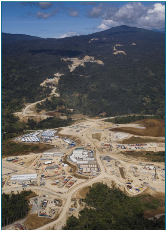
Hides Gas Conditioning Plant and Hides well pad access road
