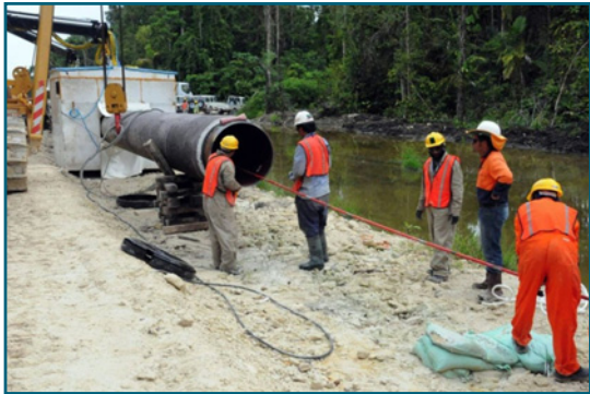
Pipe welding team
