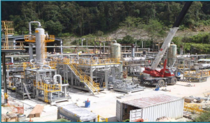
TEG Dehydration Unit installation
