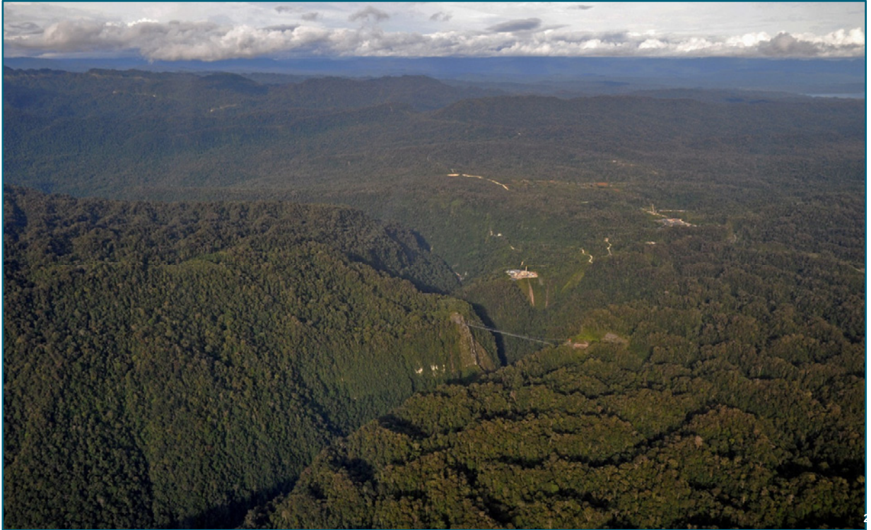
Moran, SE Mananda, Agogo 6 wellsite & Agogo Production Facility
