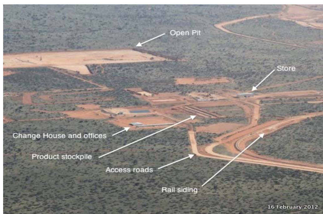
Tshipi Borwa site aerial photo
