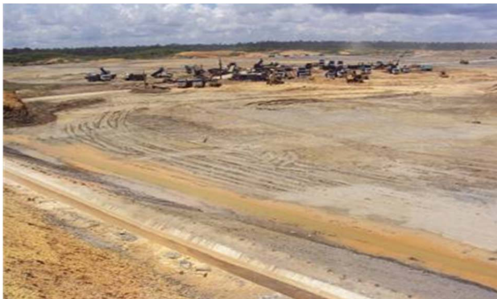
Earthworks at the OM Samalaju Site
