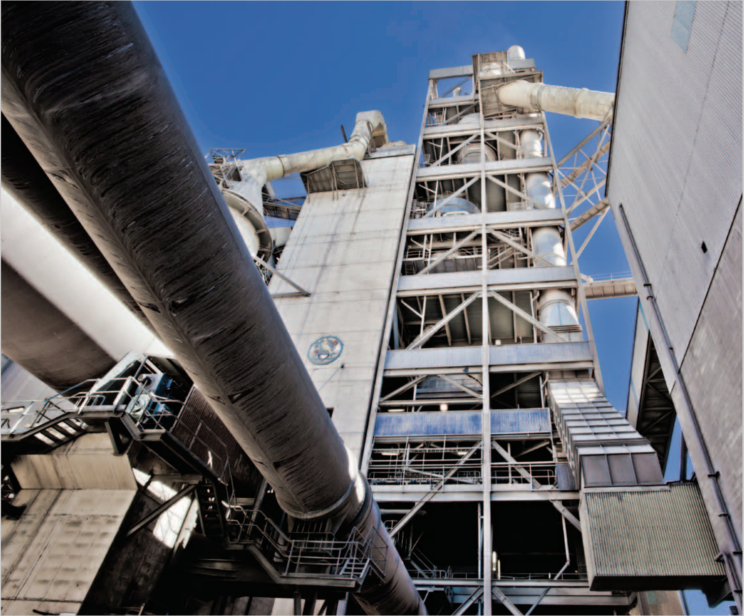
Birkenhead plant, South Australia
