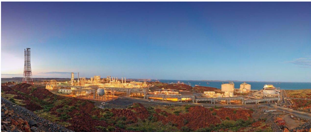
The Pluto LNG plant and associated infrastructure.
