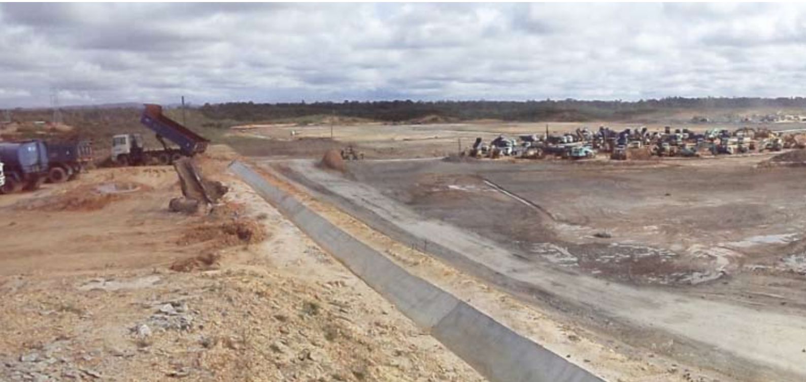
Earthworks at the Sarawak site
