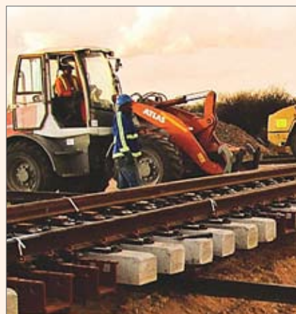
Rail Siding Construction
