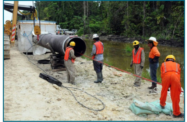
Pipe welding team
