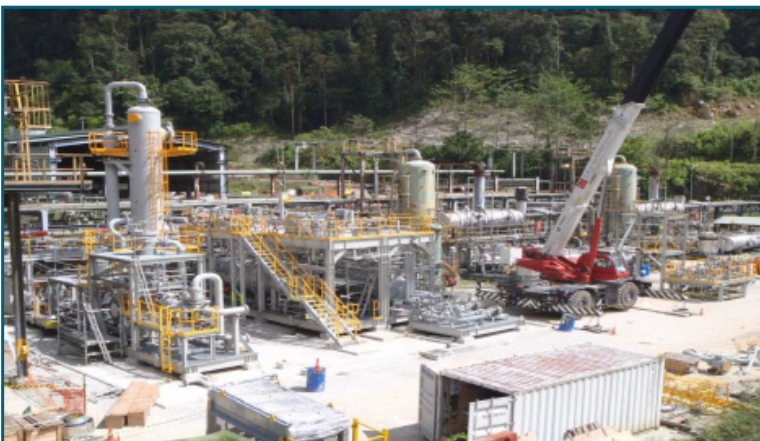
TEG Dehydration Unit installation
