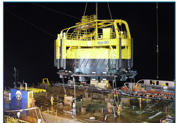
New CALM Buoy being lowered into position – first offtake March 2012
