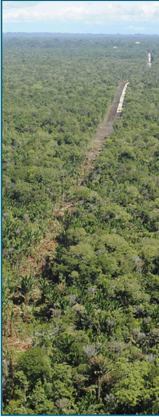
Pipeline route clearing
