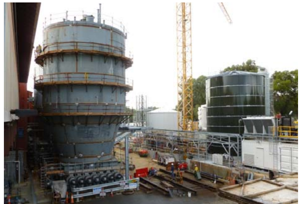
4. Side view of DiCOM vessel with anaerobic liquor tank
