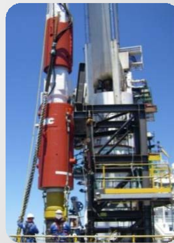
Boat Installed Conductor Production Acceleration
