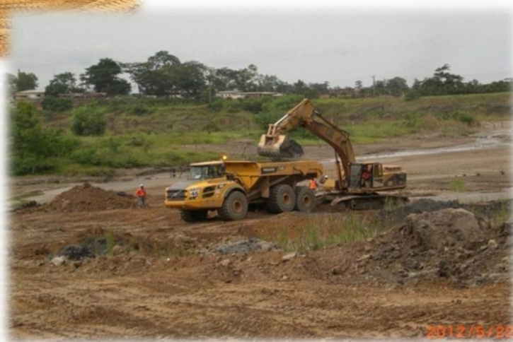
Old Tailings recovery operation – Dam 2
