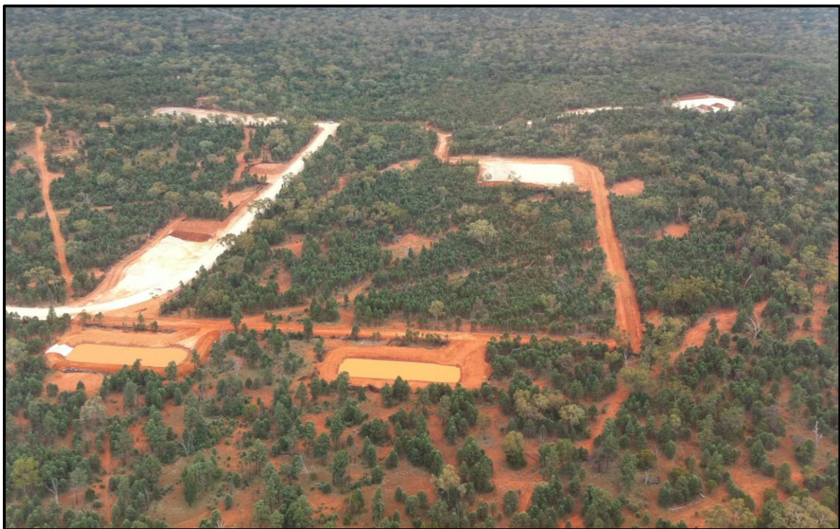
Stage 1 Earthworks completed at Hera – April 2012
