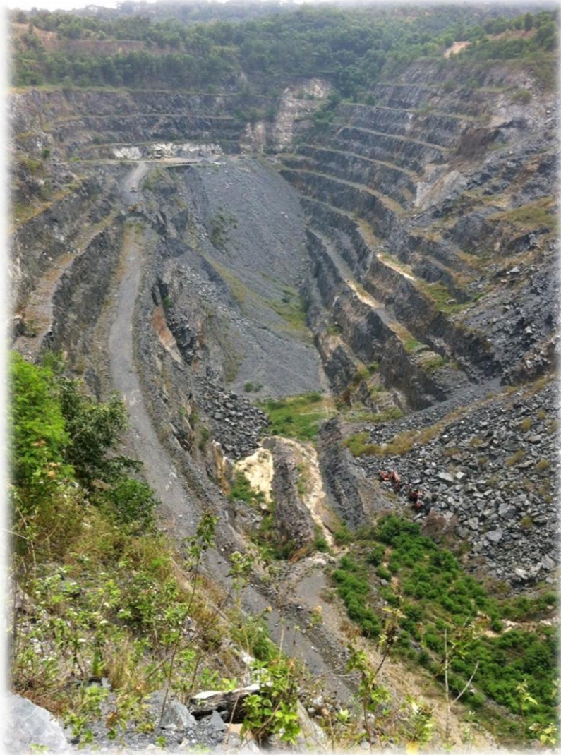
Bibiani Main Pit – looking south
