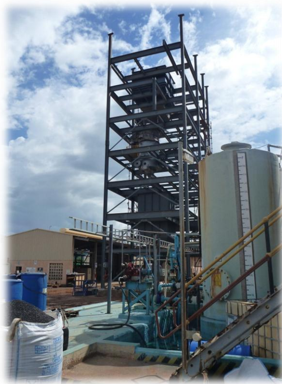
Carbon regeneration kiln Source: BBY 22/06/2012
