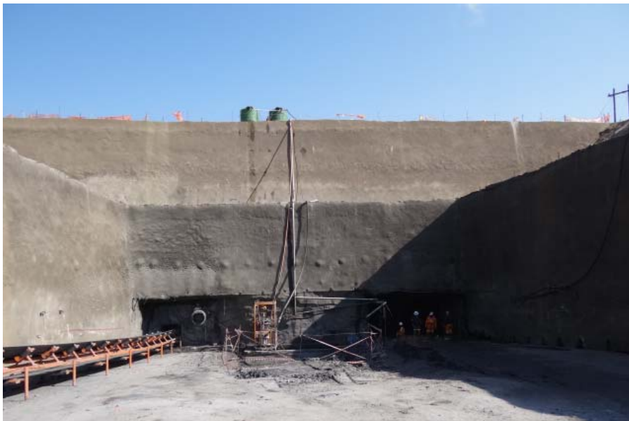
The Box-Cut of the Penumbra Coal Mine with the Conveyor Decline and Travelling Roadway
