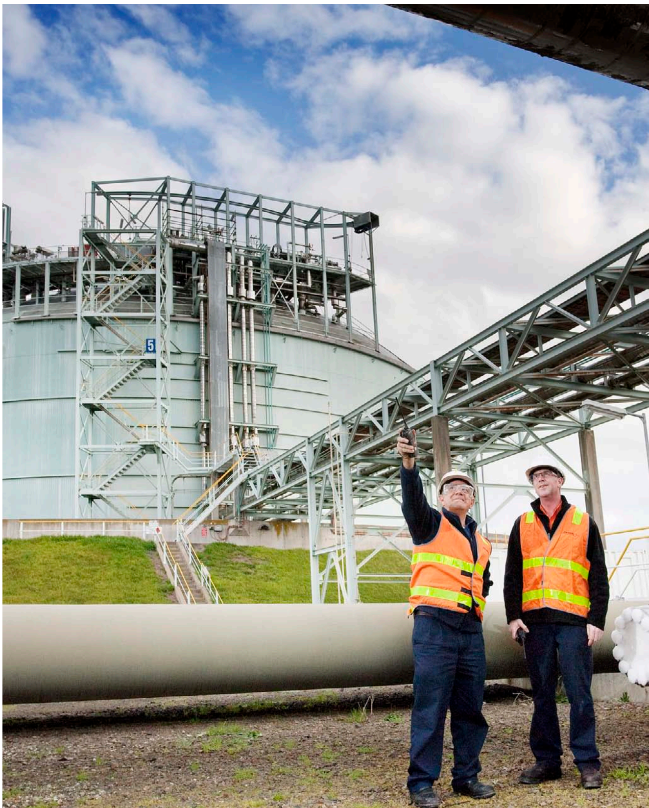
Dandenong LNG storage facility, Victoria
