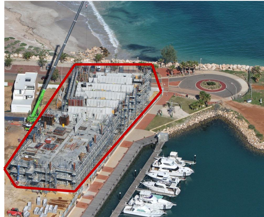
Apartments under construction at the Geraldton marina
