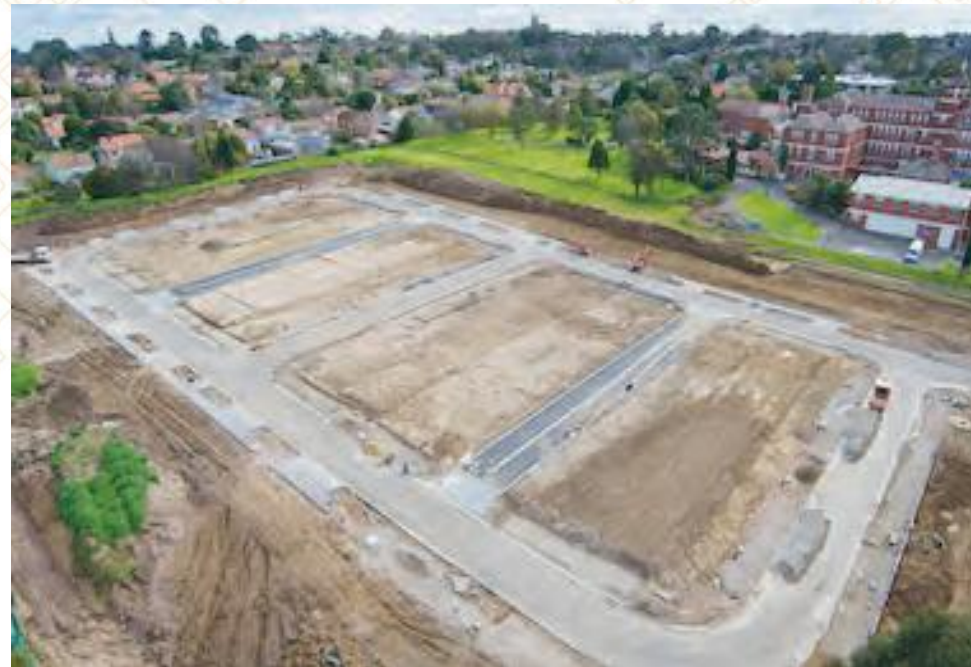
Construction of first phase to commence 1Q FY2013
