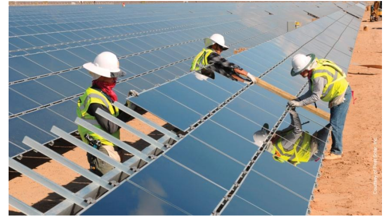
Workers installing modules at Blythe Solar Plant, California, 21 MW
