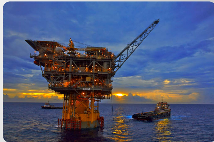
The Neptune tension leg platform in the Gulf of Mexico
