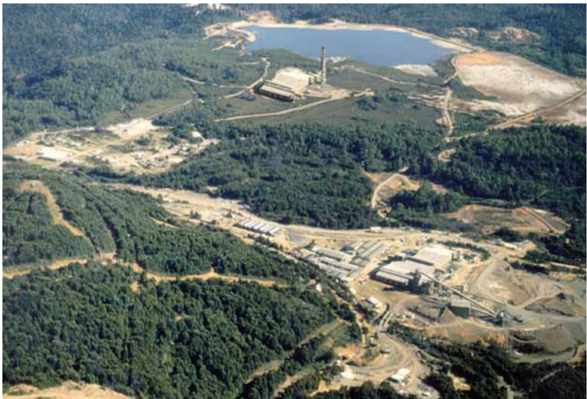
Plate 3. Aerial photograph showing conceptual Rentails Fumer in background with existing Processing Plant and Tailings Dam
