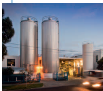
COBURG 10-16 Allenby Street Coburg VIC 3058 Australia
