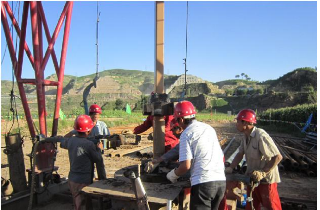
Drilling commencing at LXSG-05
