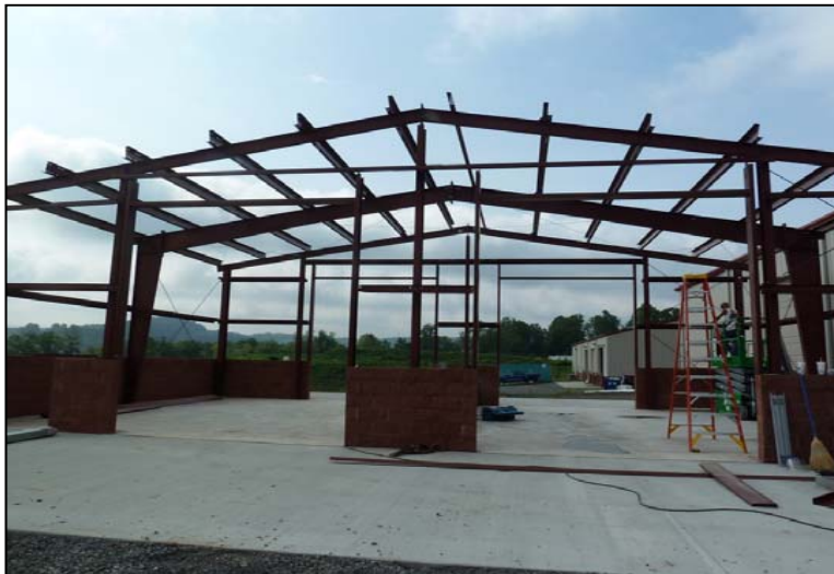
Coal Preparation Shed
